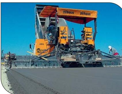
**Asphalt type paving equipment is used to place RCC pavement at the Hyundai auto manufacturing facility in Montgomery, Ala.**
